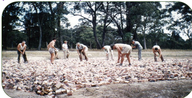
Figure 1 Laying foundations for another green 1960 ( L-R) J.Rimington, C Mayne, P Coad, J Bailey, R Case, G Williamson (Four unknown) (Photo BGC)
