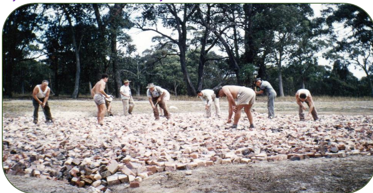
Figure 1 Laying foundations for another green 1960 ( L-R) J.Rimington, C Mayne, P Coad, J Bailey, R Case, G Williamson (Four unknown) (Photo BGC)
